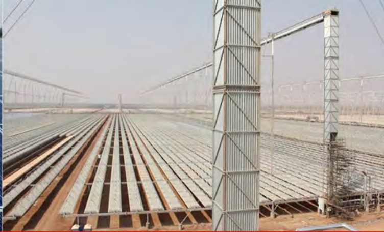
Concentrated Solar Power Plant in Rajasthan
